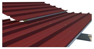
Complete the overlapping phase by positioning panels one at a time, making sure that they are correctly fixed with screws.
